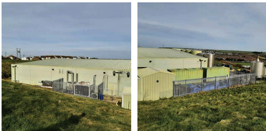
Photos of the former Arla Creamery building and landscape bund to the front of image
