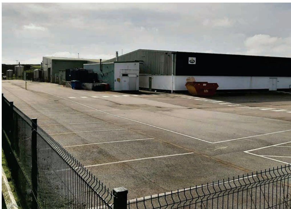
Existing building showing the extensive car park and service yard
